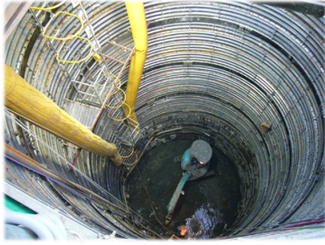
Pit for caisson type pile foundation
