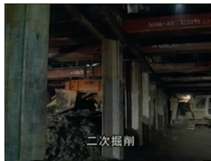
scraping by bulldozer
