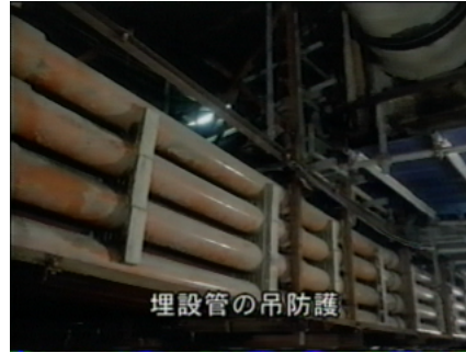
temporary supports for buried pipes
