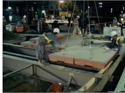
placing deck plates
