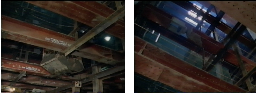
Lifting excavated soil by crab shell
