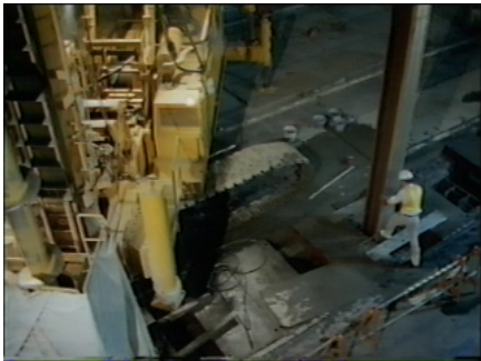
Installing a king pile
