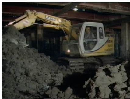
excavation by backhoe
