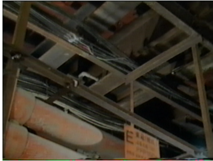
temporary supports for buried pipes
