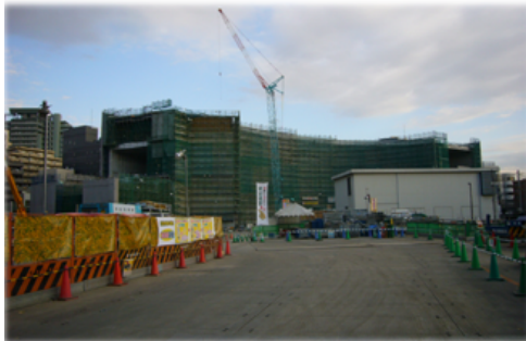
Super-structure of loop roadways of the JCT
